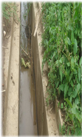
Figure 7. Modern concrete irrigation canal made in Cembe, Adola Rede District, not cleaned and know stop giving service.
